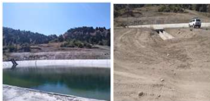
Figure 7. A reservoir to collect mudflow water
