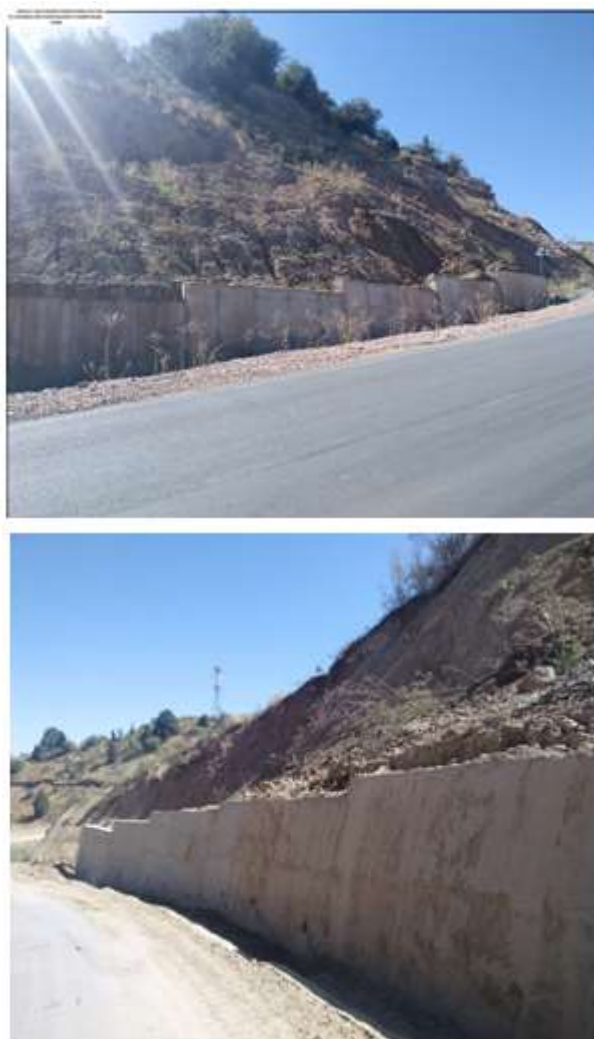
Figure 4. The protection wall was filled with sliding rocks and surpassed some parts
