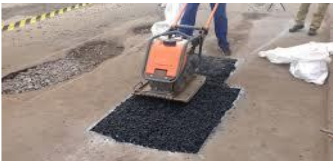
Figure 2 Road section under repair in our country
