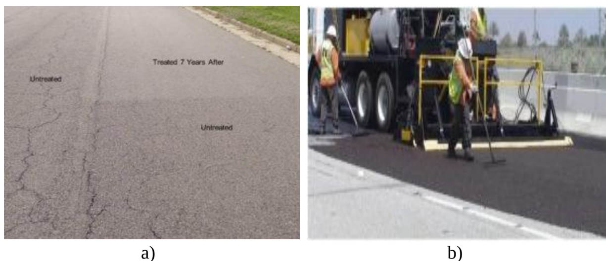
Figure 1 Renovation of the road pavement system of European countries a) before renovation b) during renovation
